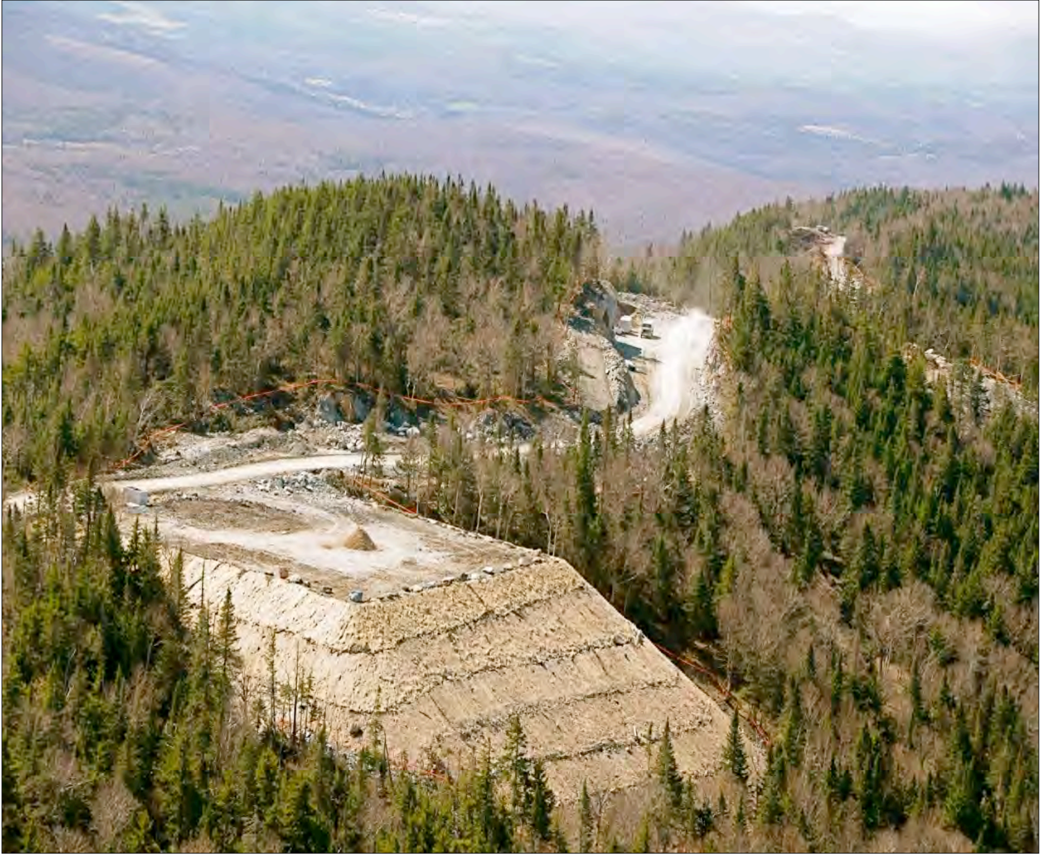
One of Twenty-One Wind Turbine Pads, Lowell Mountain, Vermont Photo by Steve Wright
