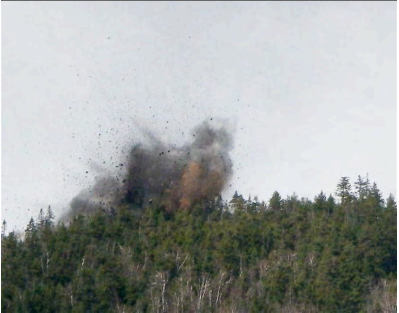
Uncontrolled Blasting, Lowell Mountain, Vermont
