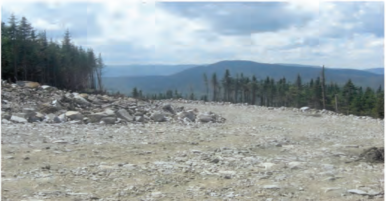
Same Roadway After Blasting on Way to Mt. Kelsey
