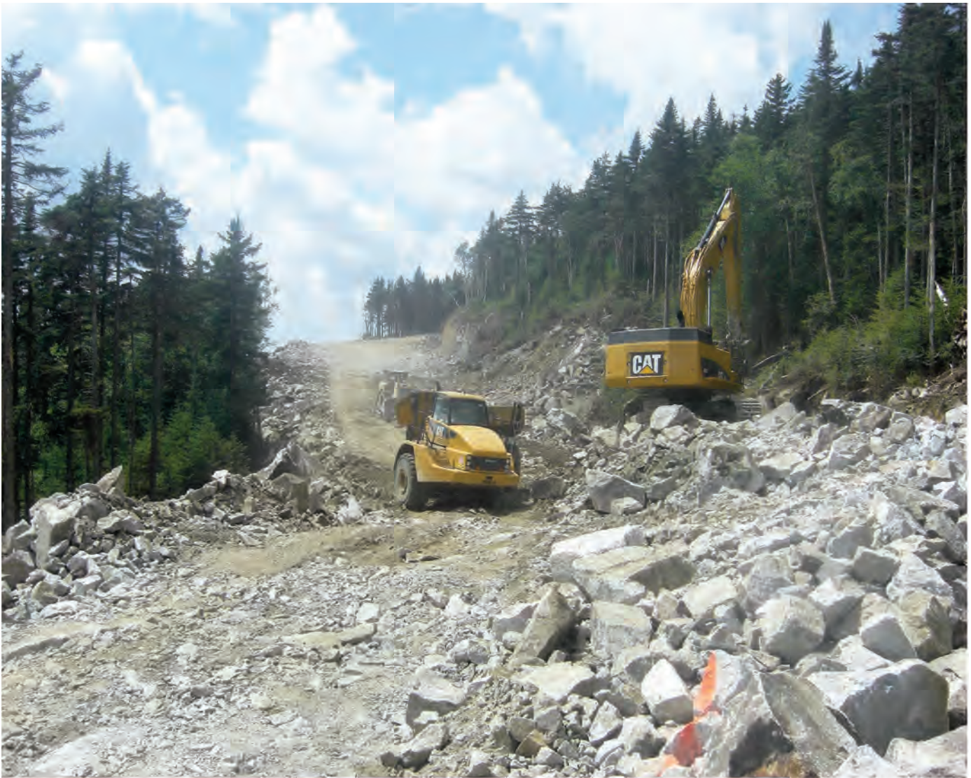
Road to Mt. Kelsey After Blasting
