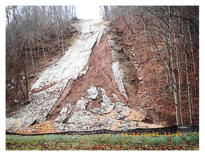
This photo from West Virginia regulators shows the failure of erosion controls.
