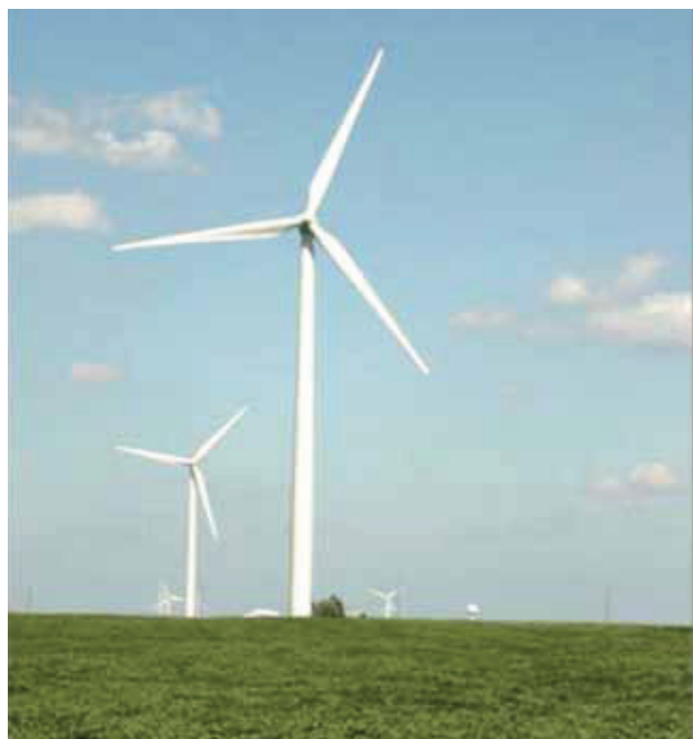
Utility-scale wind turbines located in Huron County, Michigan.
