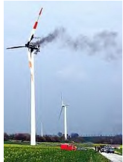
Figure E.6.1: Turbine fire in east Germany. Fire brigade has cordoned off the area to allow the fire to burn out.
