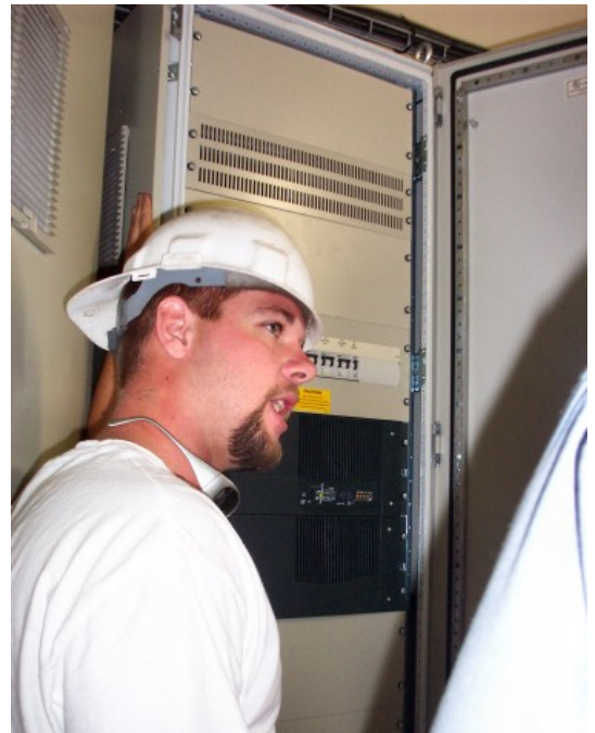
Figure C.1: Chris, a Vestas employee, explains how remote monitoring works while inside the turbine.
