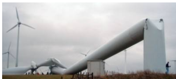
Figure E.9.2: Structural failure in western Germany.
